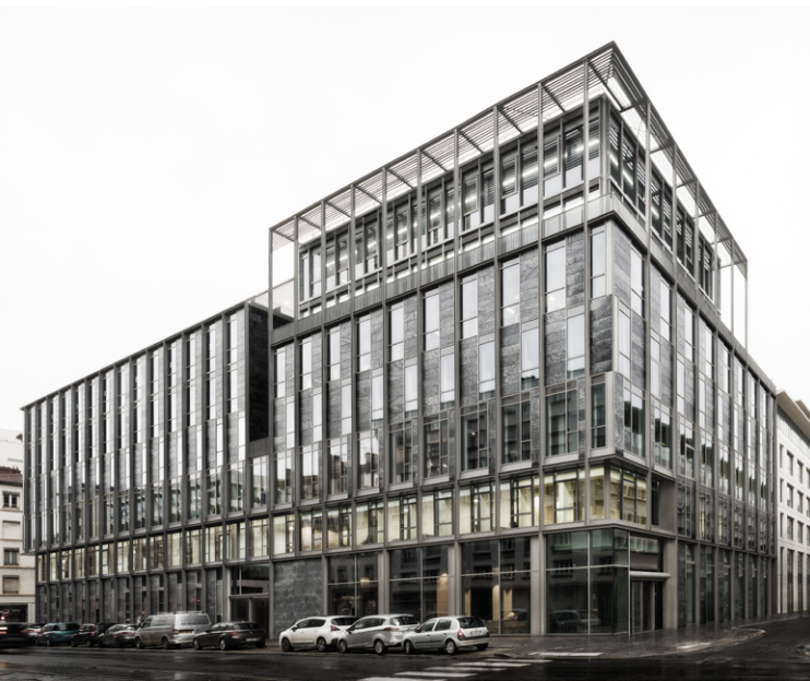
COLEGIO ABOGADOS LYON / OFFICE OF ARCHITECTURE IN BARCELONA (OAB)
