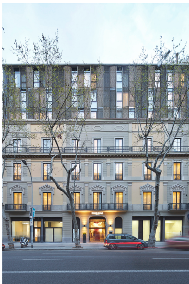
HOTEL VINCCI GALA EN BARCELONA / TBI ARCHITECTURE & ENGINEERING
